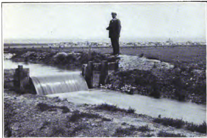
WOODEN MEASURING WEIR IN LATERAL CANAL, WILLISTON, NORTH DAKOTA.
